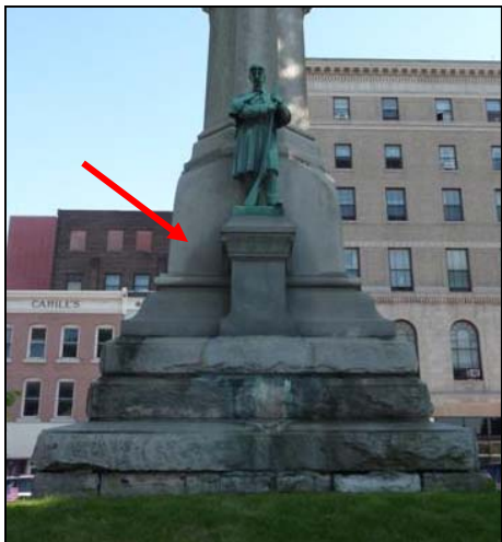
Figures 13-15. The stone exhibits some unevenness of color due to variations in weathering (left and center), leaving some minerals more exposed (detail, right).
