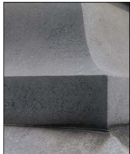
Figures 13-15. The stone exhibits some unevenness of color due to variations in weathering (left and center), leaving some minerals more exposed (detail, right).
