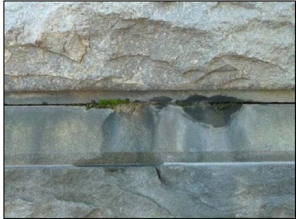
Figures 11 and 12. Soiling and biological matter has accumulated in the recesses approaching joints (left), and in joints which remain damp.
