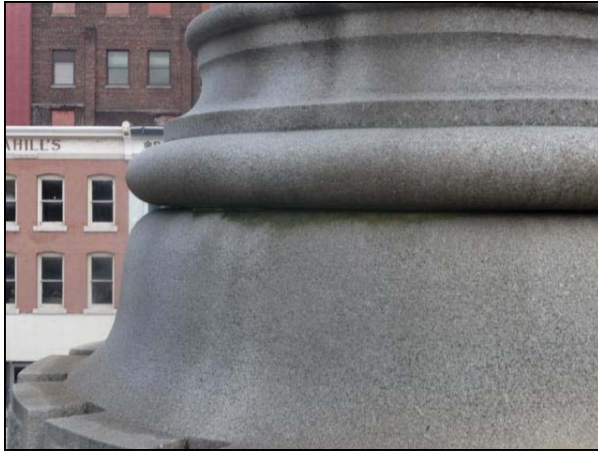
Figures 11 and 12. Soiling and biological matter has accumulated in the recesses approaching joints (left), and in joints which remain damp.
