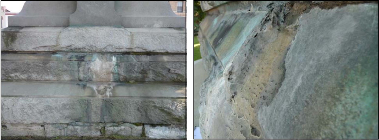
Figures 19 and 20. Overall (left) and detailed image (right) of the dense calcite run which has developed on the north elevation of the base.
