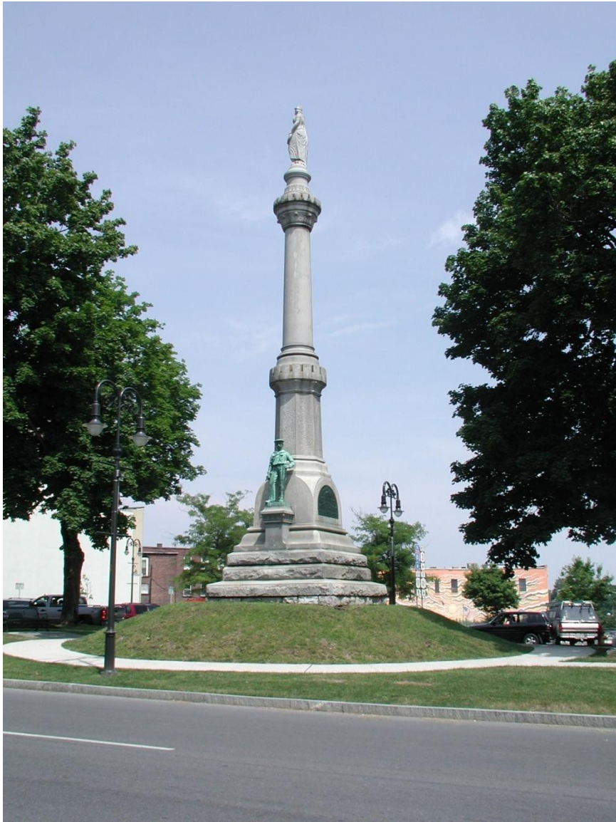
Photo 1. View of the Soldiers and Sailors Monument from the South side.
